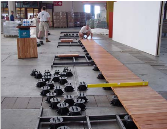
EXHIBITION FLOORING - BUZON PEDESTAL & TILE COMBINATION
